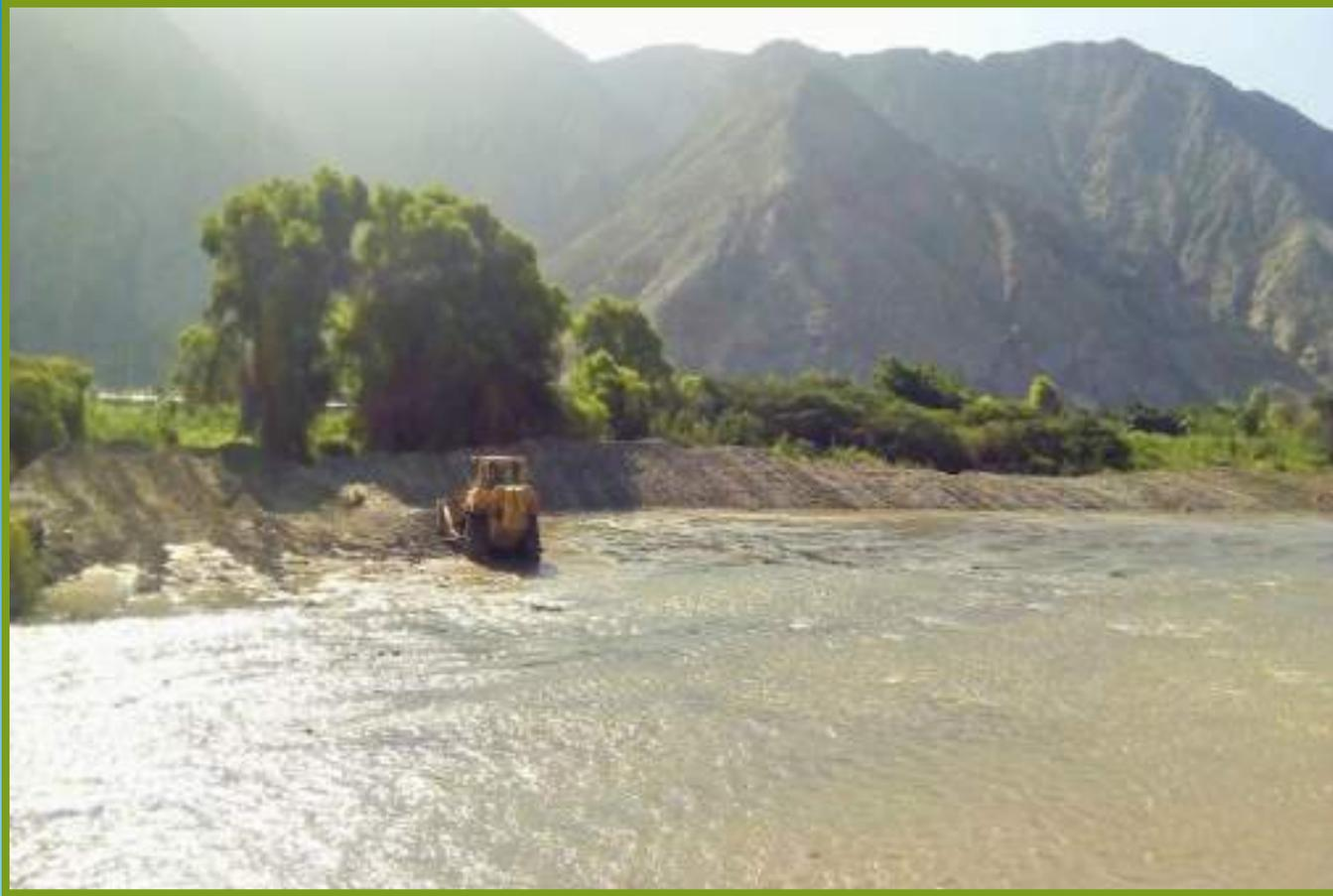
**FOTO 05:** CORTE Y ARRIMADO DEL MATERIAL DEL CAUCE
