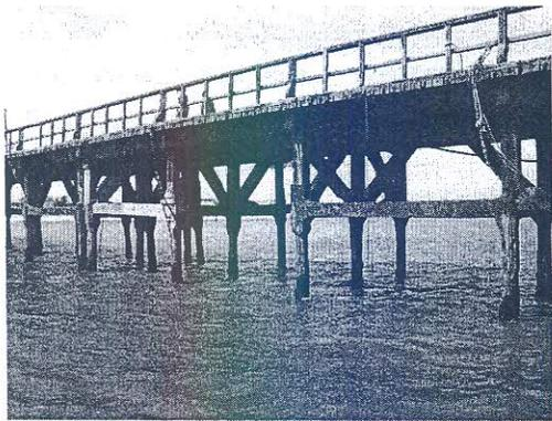
CONCRETO DESPRENDIDO DEBIDO A LA CORRSION DEL ACERO
