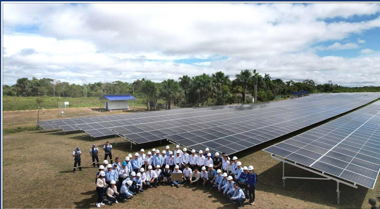
Central Solar San Lorenzo 3 MWp / 2MWh
