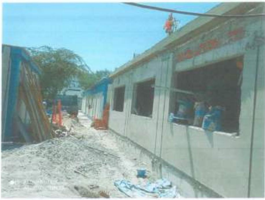
TARRAJEO EN MUROS EXTERIORES C/MEZCLA C:A 1:5 E=1.5CM
