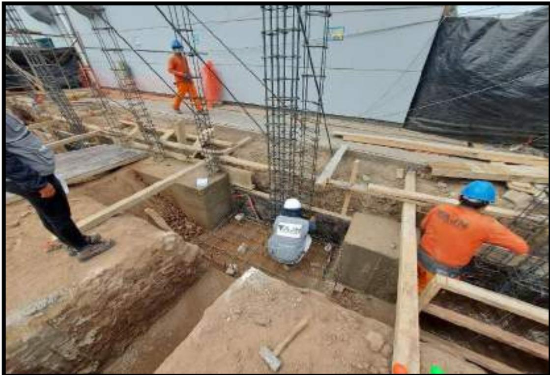
VERIFICACION DE ARMADURA DE ZAPATAS, ANCLAJE DE ARMADURA DE COLUMNAS EN EL EJE D-D
