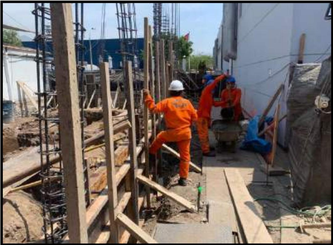
COLOCACION DEL CONCRETO F'C=100KG/CM2 EN SOBRECIMIENTO DEL EJE D-D
