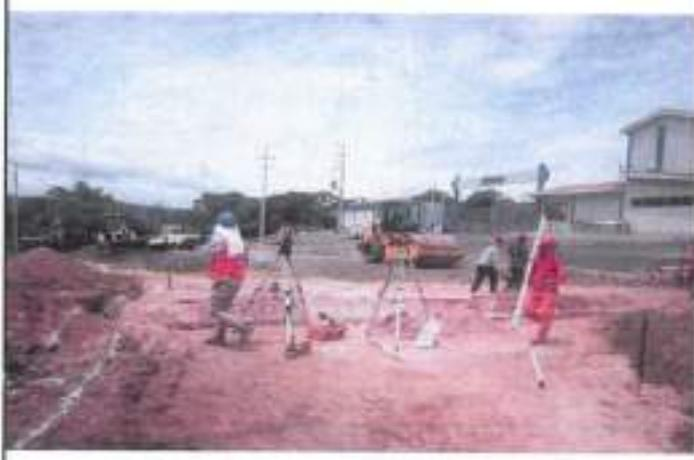
**FOTOGRAFIA 01:** TRAZO, NIVELES Y REPLANTEO DURANTE EL PROCESO.
