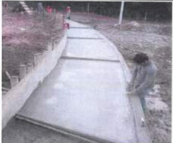
**FOTOGRAFIA 06:** CONCRETO PREMEZCLADO DE  $f_c=175$  kg/cm<sup>2</sup> EN VEREDAS. ACABADO SEMIPULIDO
